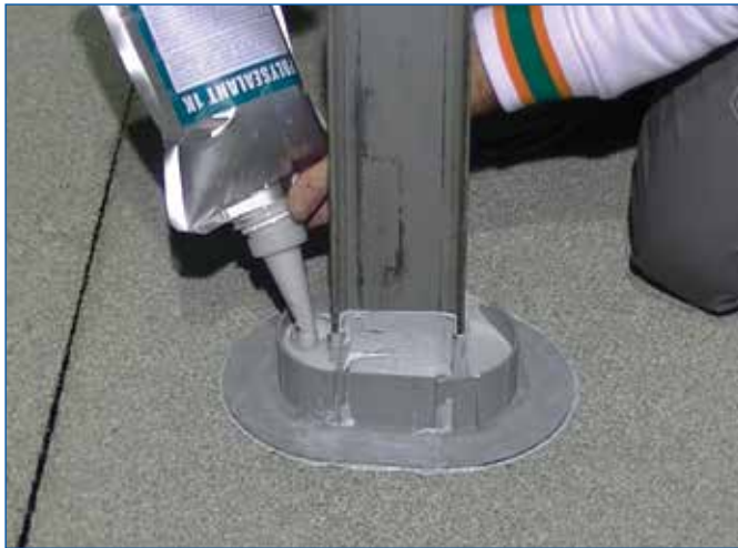
FIGURE 6 - Filling the POLYSEALANT MOULD formwork with POLYSEALANT 1K
