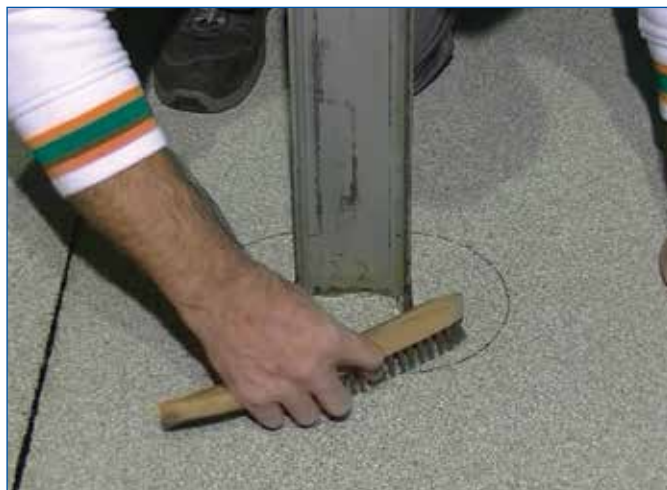
FIGURE 2 - Preparing the surfaces
