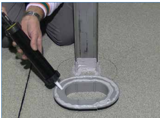
FIGURE 4 - Application of the POLYSEALANT CARTRIDGE adhesive sealant
