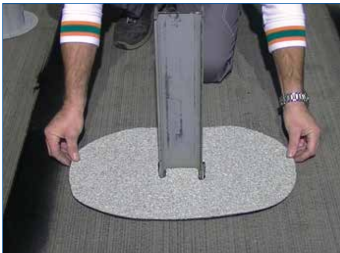
FIGURE 7 - Application of patch of mineral membrane
